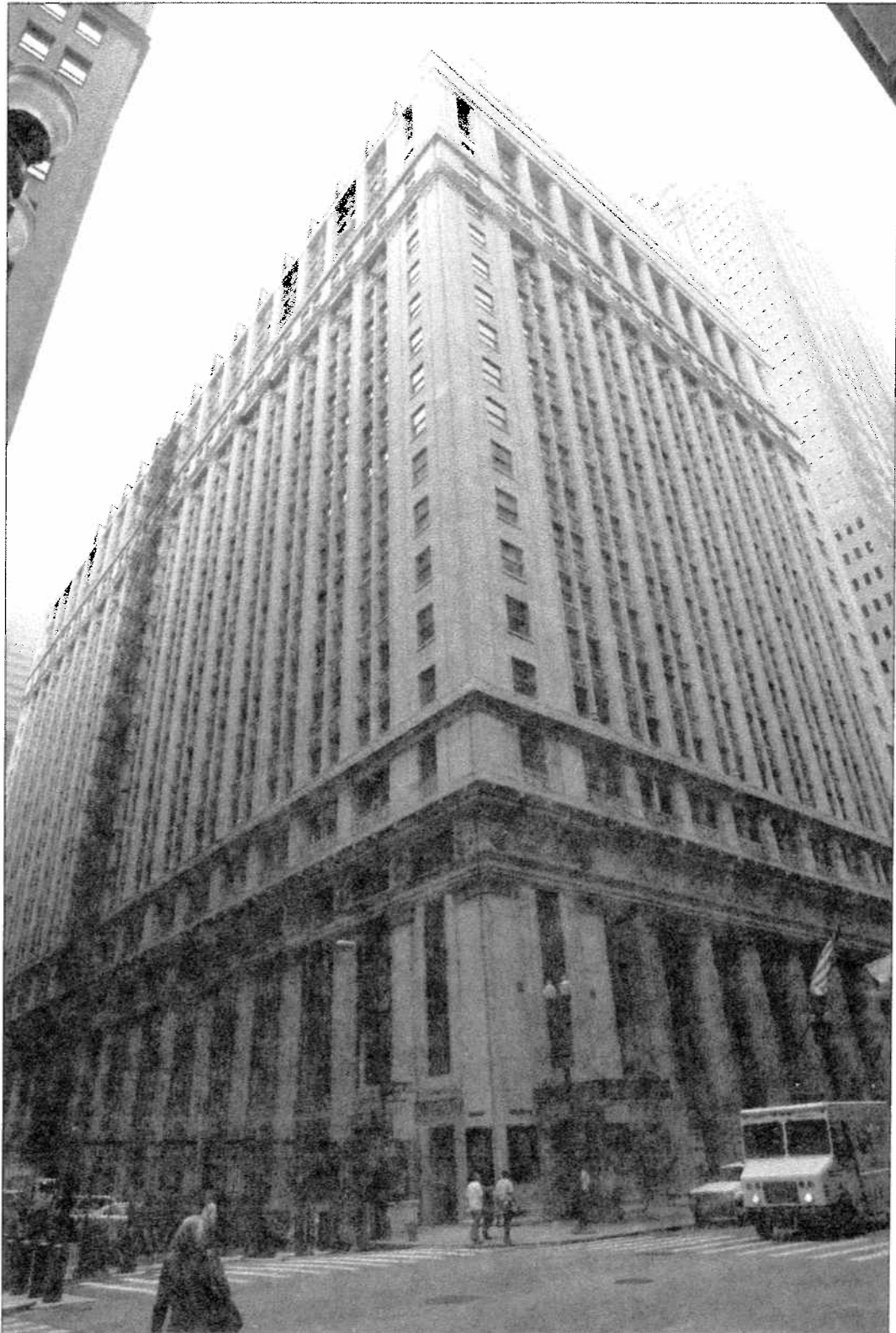
Image 43: Current photograph of the southwest corner the Continental & Commercial National Bank Building.
